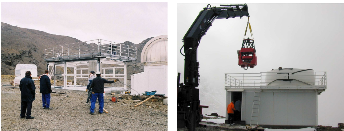
Figure 8.3: Images of BOOTES-IR during the construction of the housing during August 2003 (left) and the installation of the telescope in November 2004 (right).
